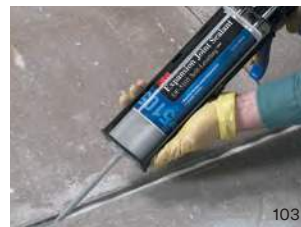
Make fast work of lengthy expansion or control joints and other larger jobs with the heavy-duty manual applicator and 12 fl oz duo-pak cartridges.
